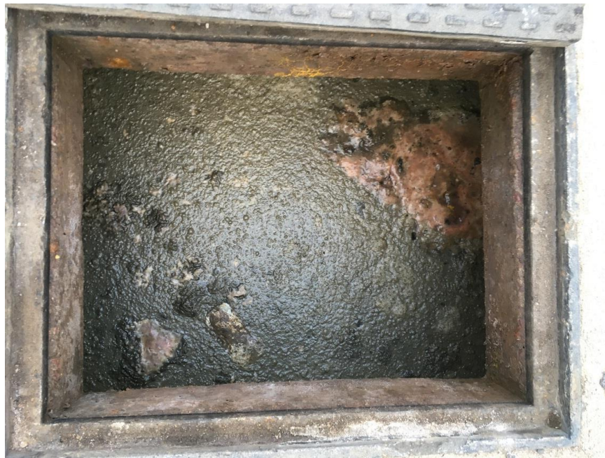
Figure A1: Scum Layer in ABR 1 of Street 3
