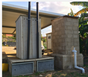
Examples of VIP latrine and composting toilet at the field site.
